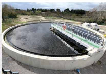
Station d'épuration (STEP)
